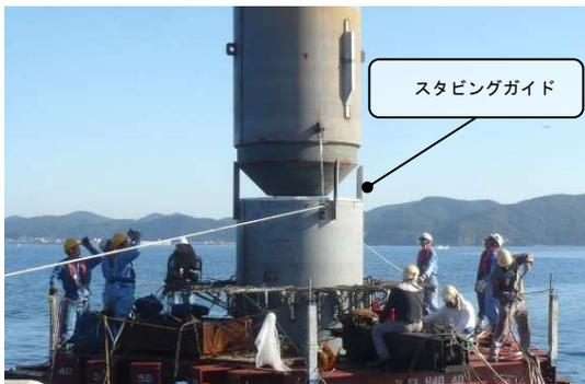
Fig. 7 Joining the upper and lower piles
