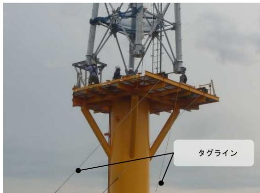
Fig. 8 lifted objects steadying control system
