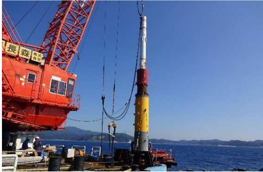
Fig. 6 Pile driving
